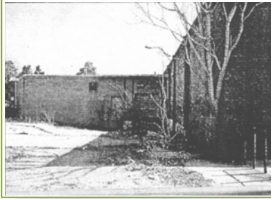
Exterior Renovation of Existing Building
