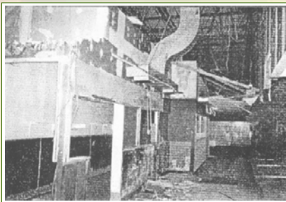
Existing Interior Conditions
